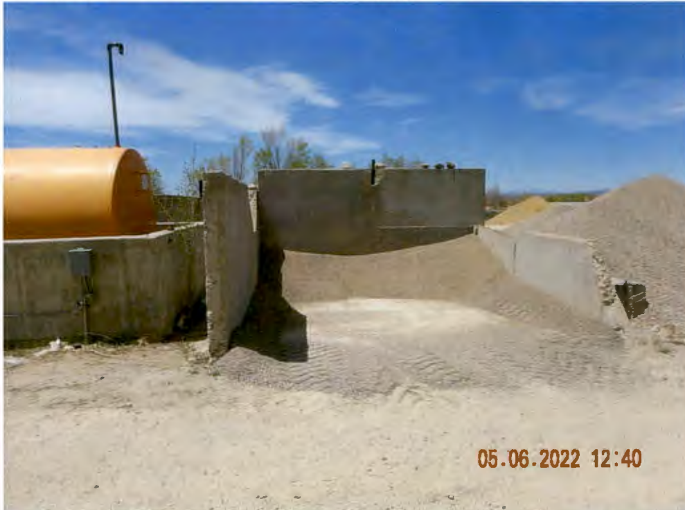
12) 3/8 " aggregate stored in 3 walled bunker near above ground diesel storage tank. Stockpile adjacent to bunker is not contained within a three walled bunker.
